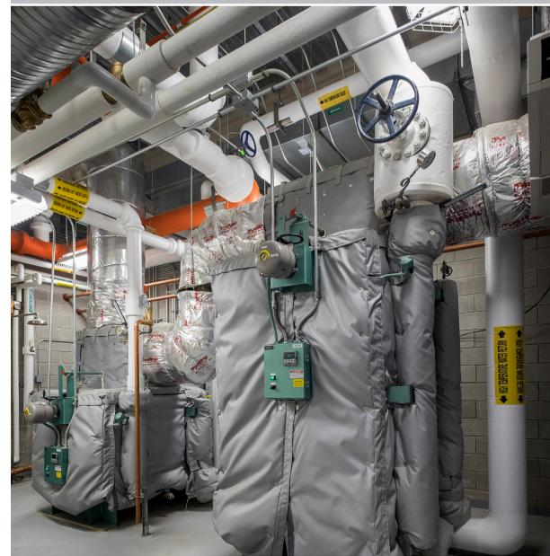
The heat exchangers transfer the exhaust heat from the micro turbines to generate hot water.
