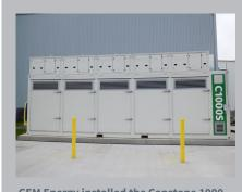
GEM Energy installed the Capstone 1000 kW Combined Heat and Power (CHP) packaged system for the facility's electrical and hot water heating needs.
